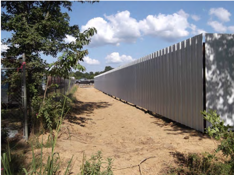
Newly Constructed fence located south of 15' Utility easement
