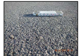
Figure 9: Weathering
