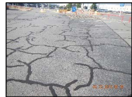
Figure 11: Block Cracking
