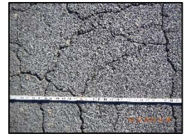
Figure 10: Alligator Cracking
