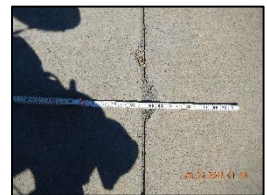
Figure 12: Joint Spalling
