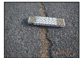
Figure 8: L&T Cracking
