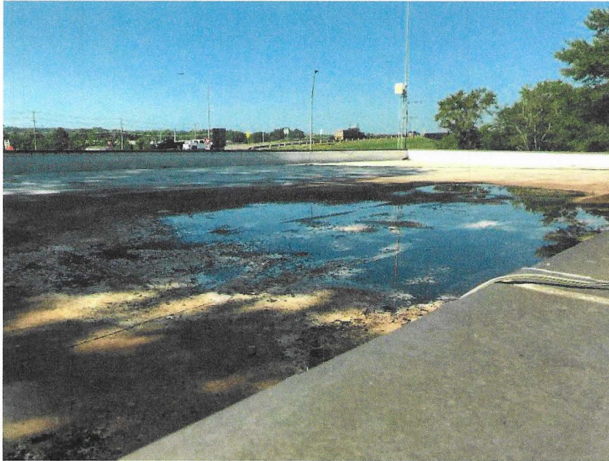
Above: Water ponding on the existing single membrane roof
