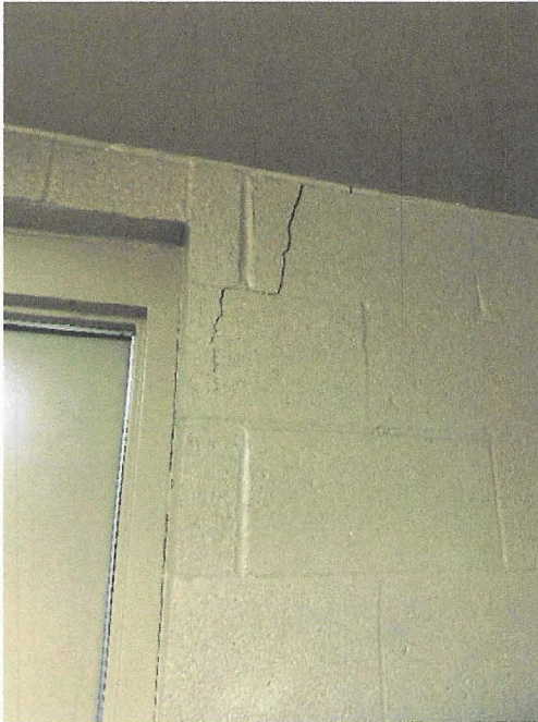
Above Left: Cracking at interior side of masonry block walls. Possibly due to heavy water penetration and surface moisture
