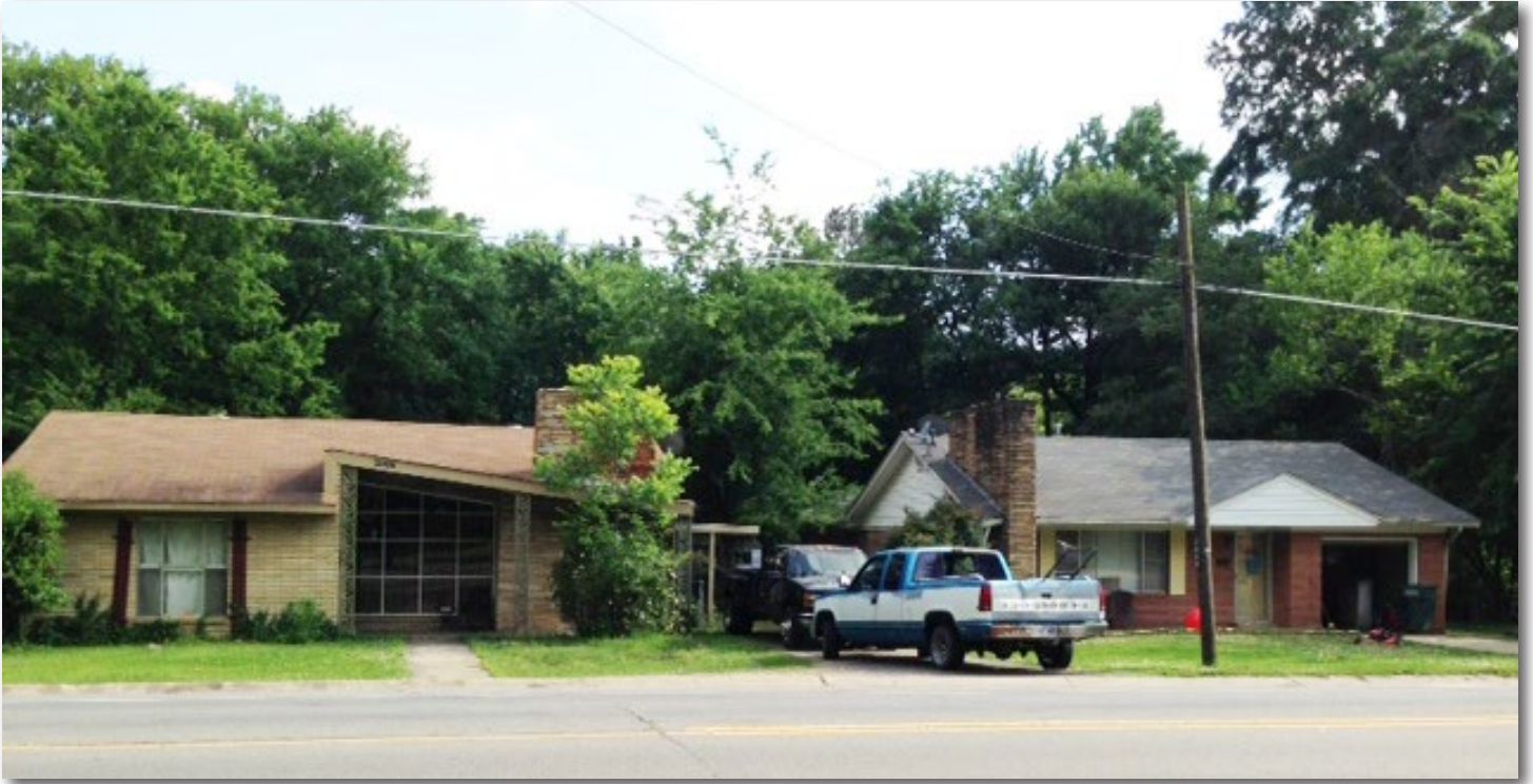
View Across Caldwell Looking South
