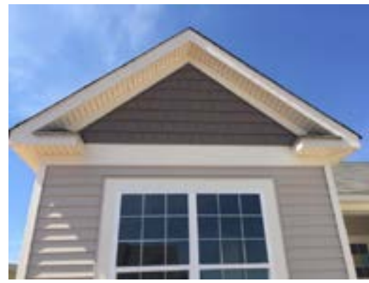
Representative trim around windows and gable end
