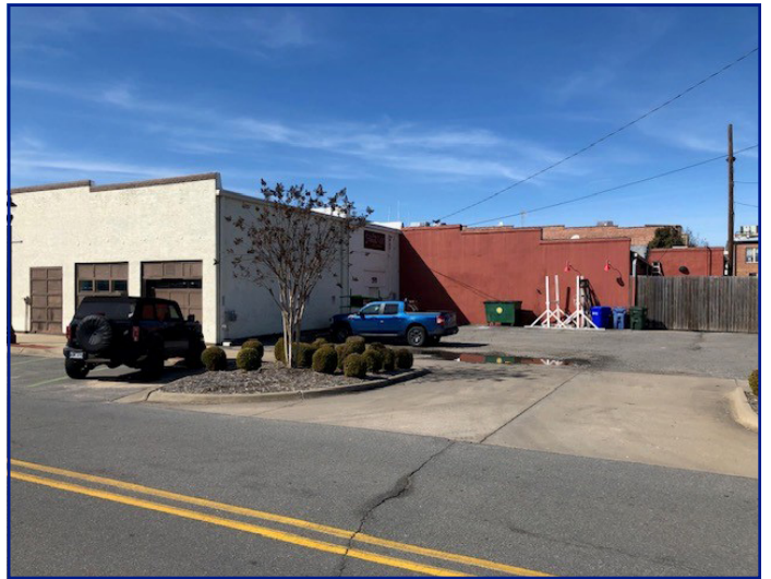
View of subject property from Main St facing NW
