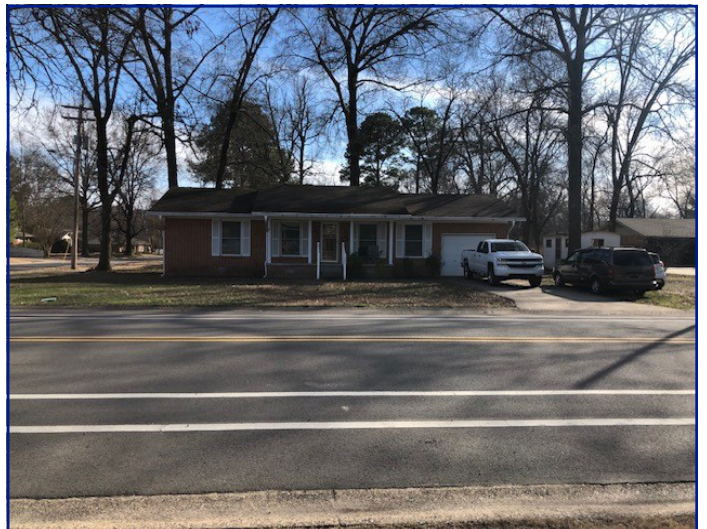
Property adjacent to the S across Robinson
