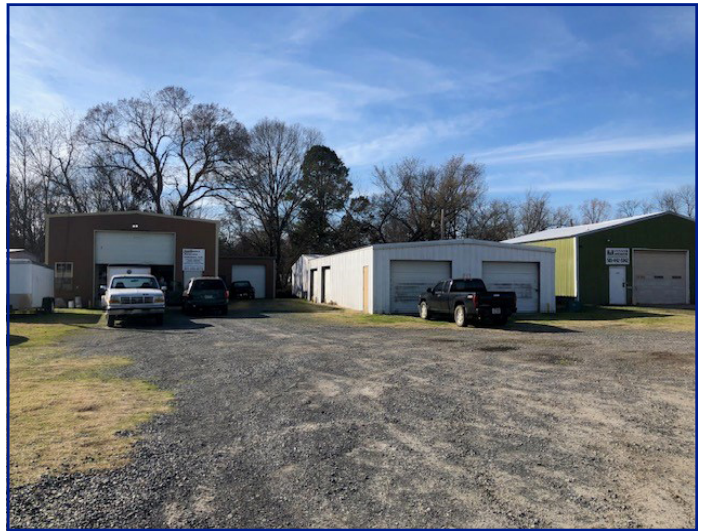
Property adjacent to the N
