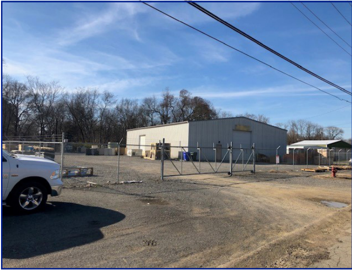
View of subject property from Parkway facing NW
