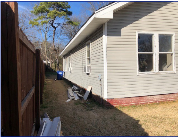
View of subject property from Prince looking NE
