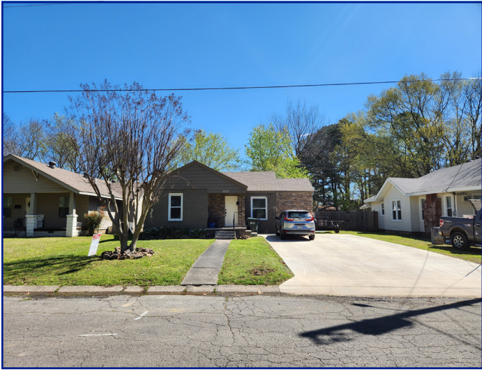
View of subject property from N Ash St facing E
