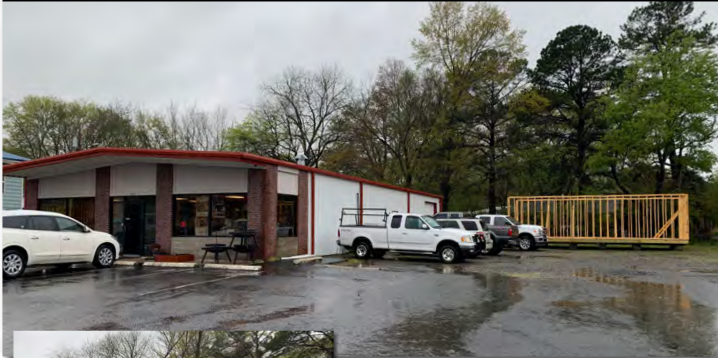
View of property looking SW
