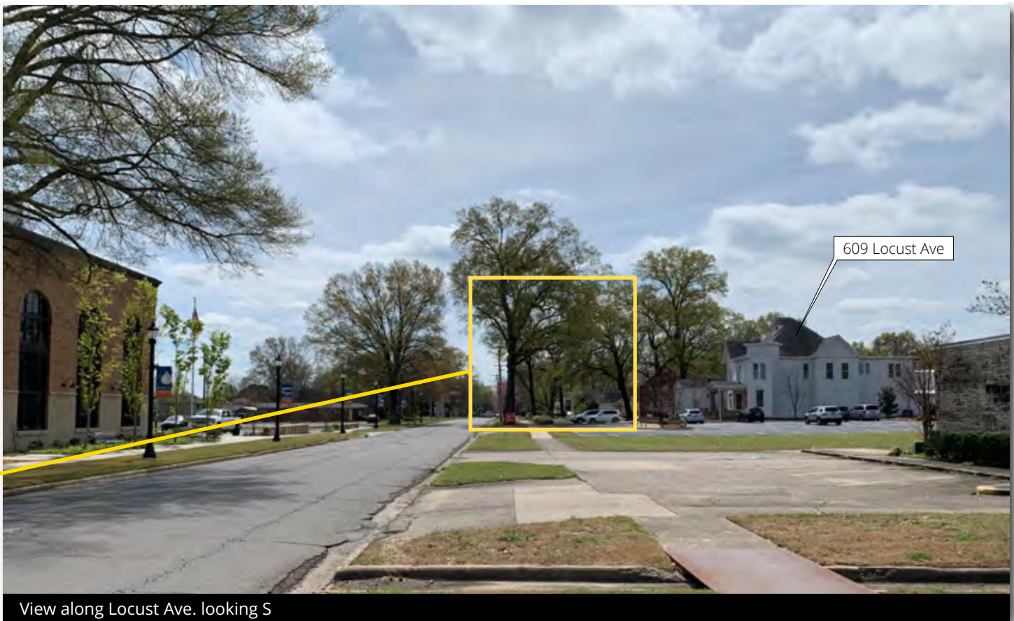
Aerial view of 609 Locust Ave.
