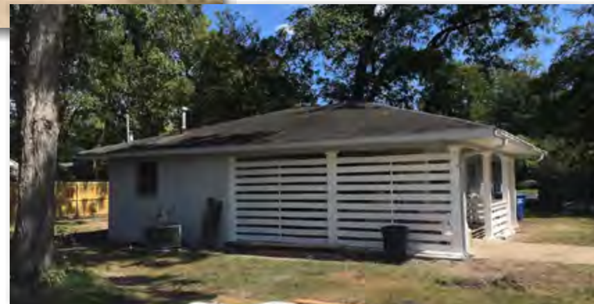
AFTER view of subject property from Robinson Ave looking northeast
