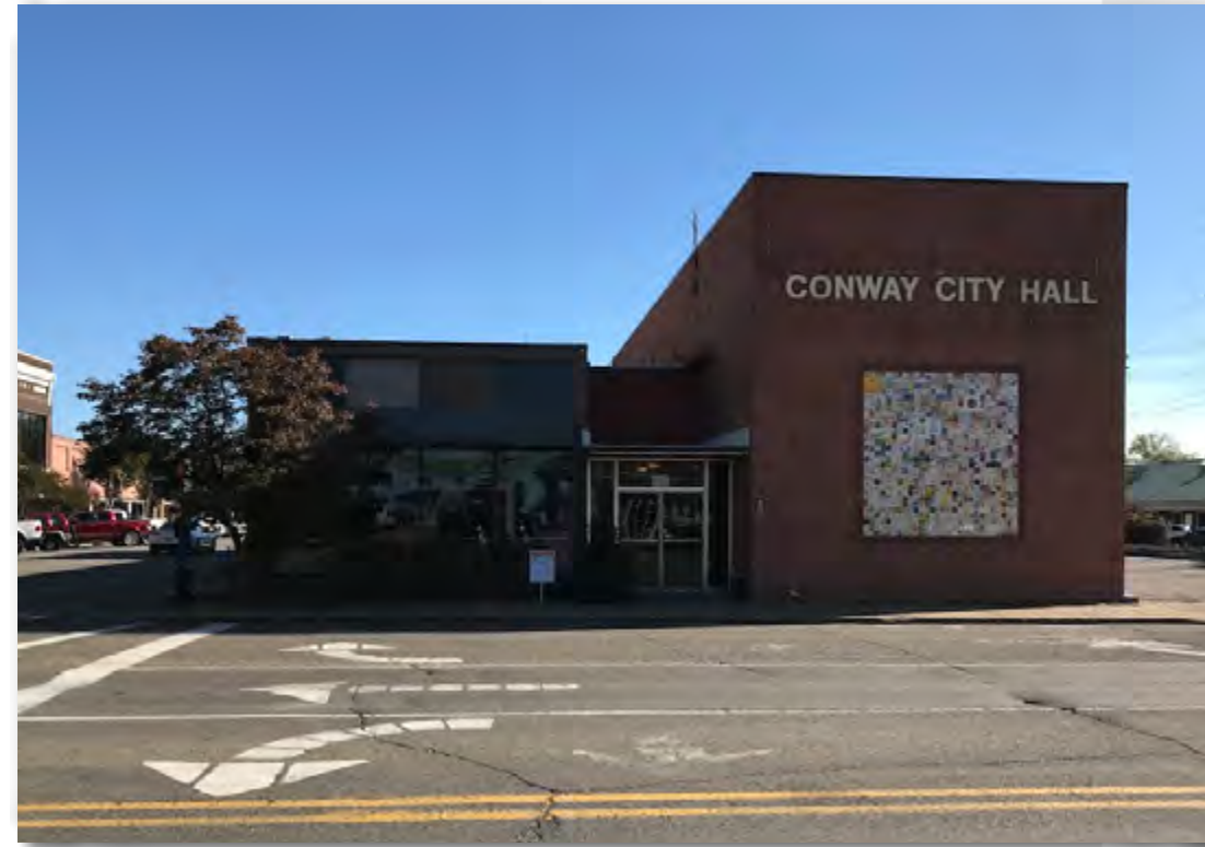
View of subject property from Oak St looking south
