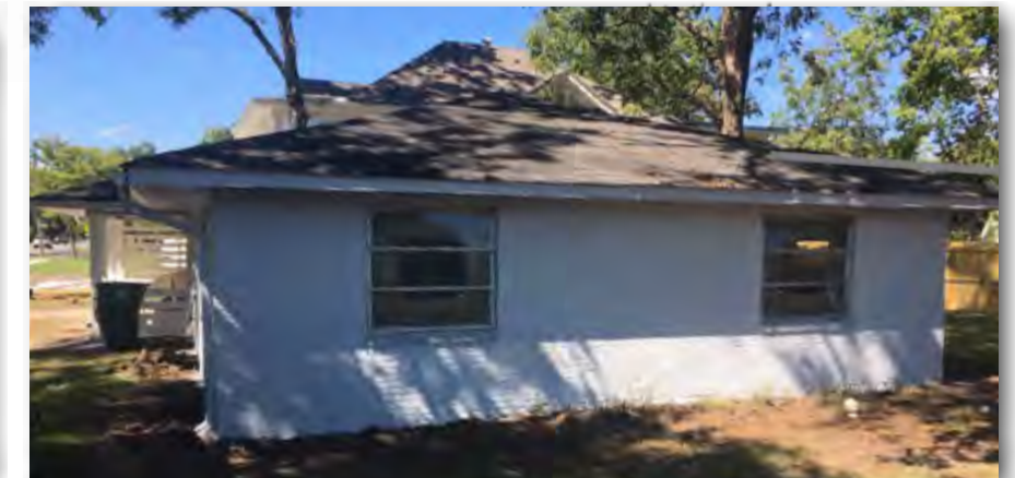
AFTER view of subject property from Robinson Ave looking west
