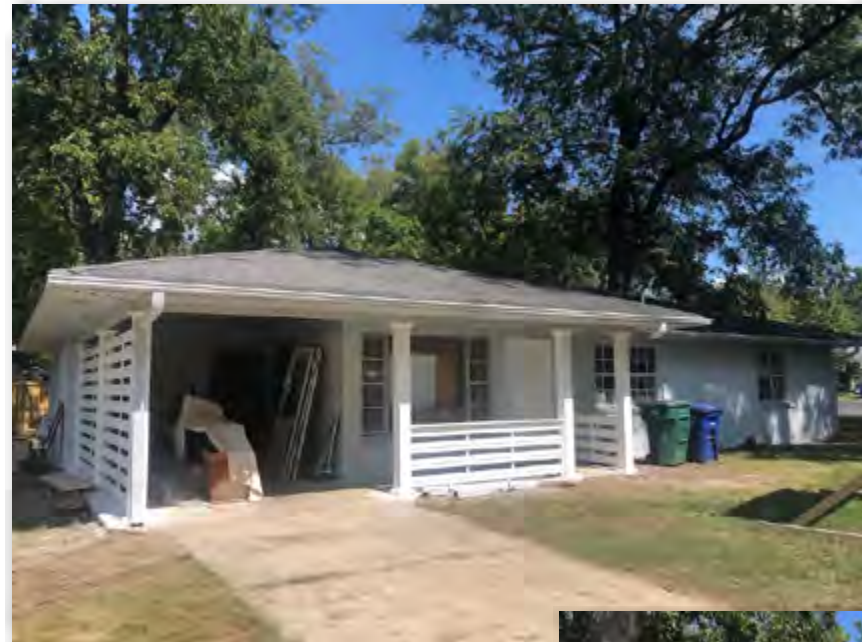
AFTER view of subject property from Robinson Ave looking northeast
