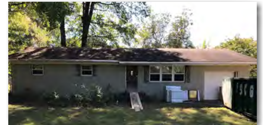
View of subject property from Independence Ave looking south
