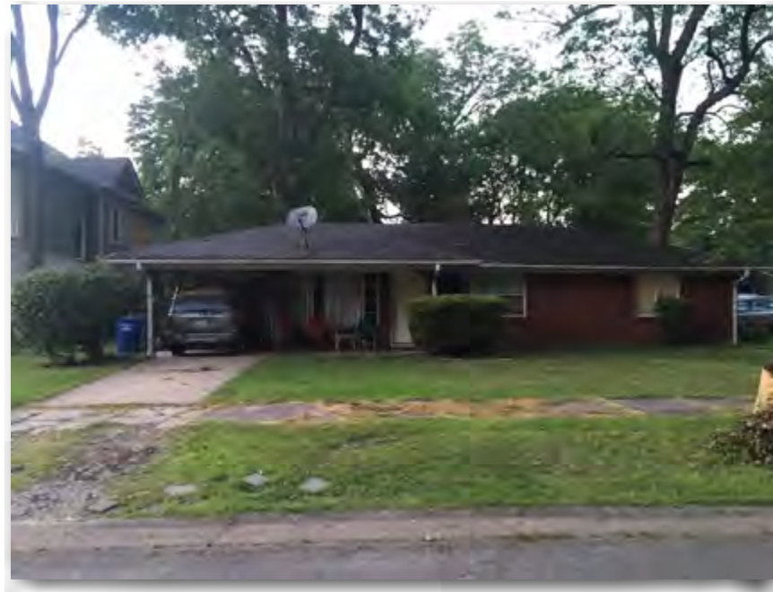
BEFORE view of subject property from Robinson Ave looking north
