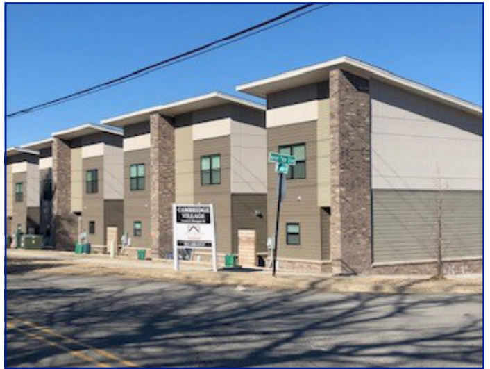
Property adjacent to the NW, across Meadowlake Rd
