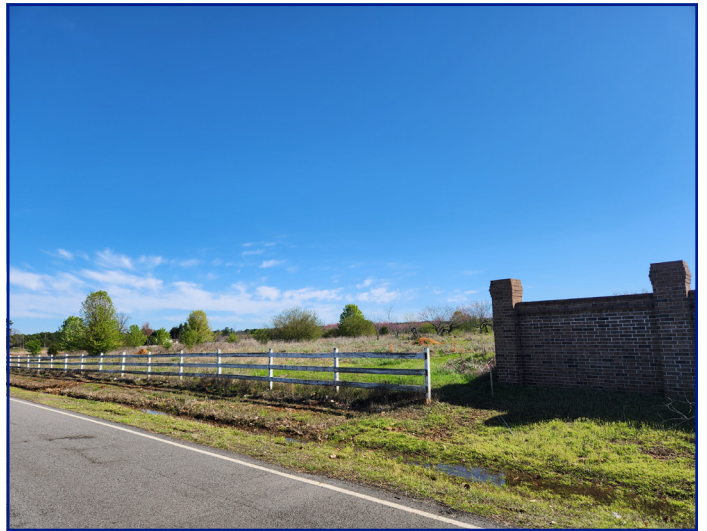
Point of contact between Phase I and Phase II
