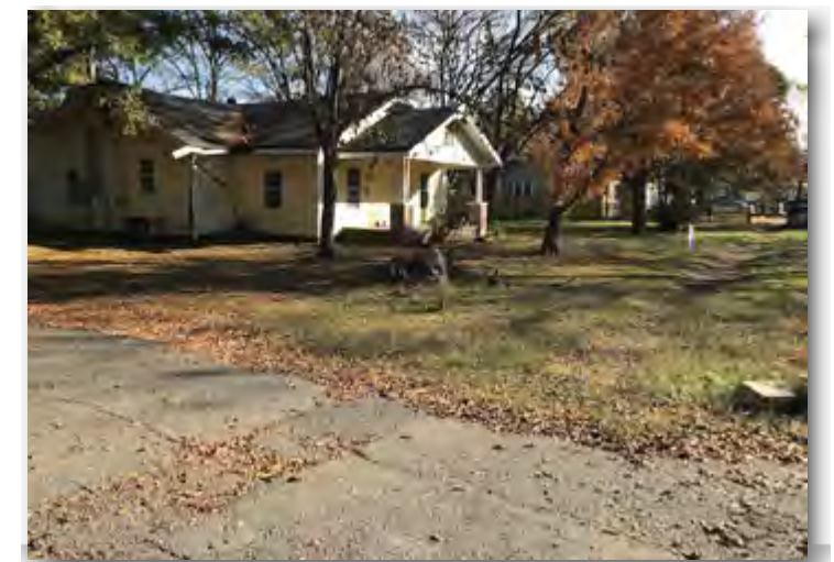
View of subject property from Ingram St looking southeast
