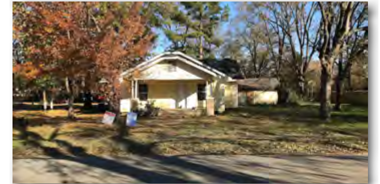
View of subject property from Ingram St looking east
