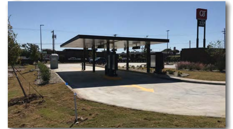
Example canopy at another location
