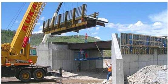
Photo 14 - Prefabricated Steel Bridge System
