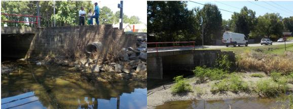
Photo 7 NE Storm Drain Thru Wingwall
